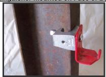
Mount Fire Extinguisher bracket on IBA-1 and tighten securely.
