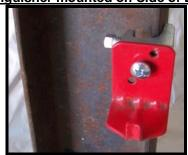
Mount IBA-1 on I-Beam or channel iron and tighten square-headed bolt.
